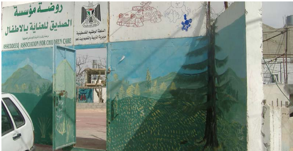
Figure (6.14): Kindergarten external walls. 1
